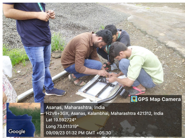
Fig 4: Students installing the Solar Street lights.
