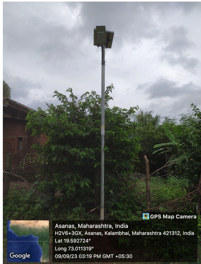
Fig 5: Solar Street light image after installation.
